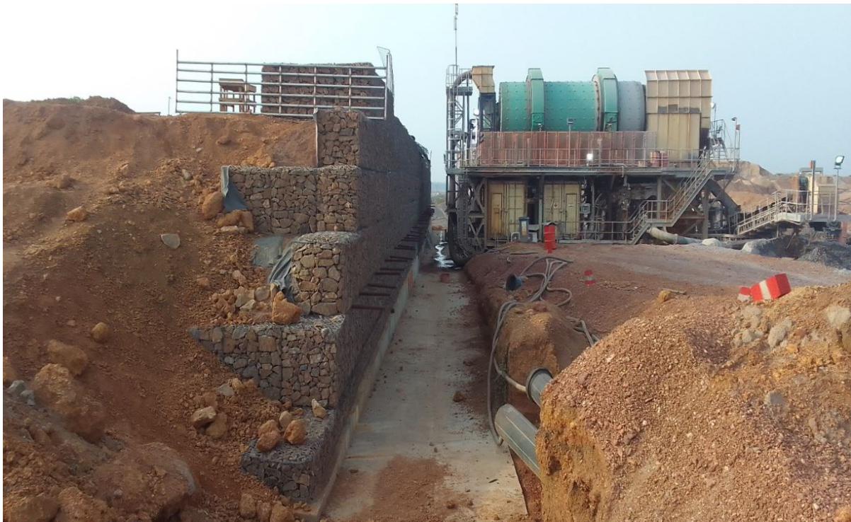
DM1/4 Gabion wall under construction
