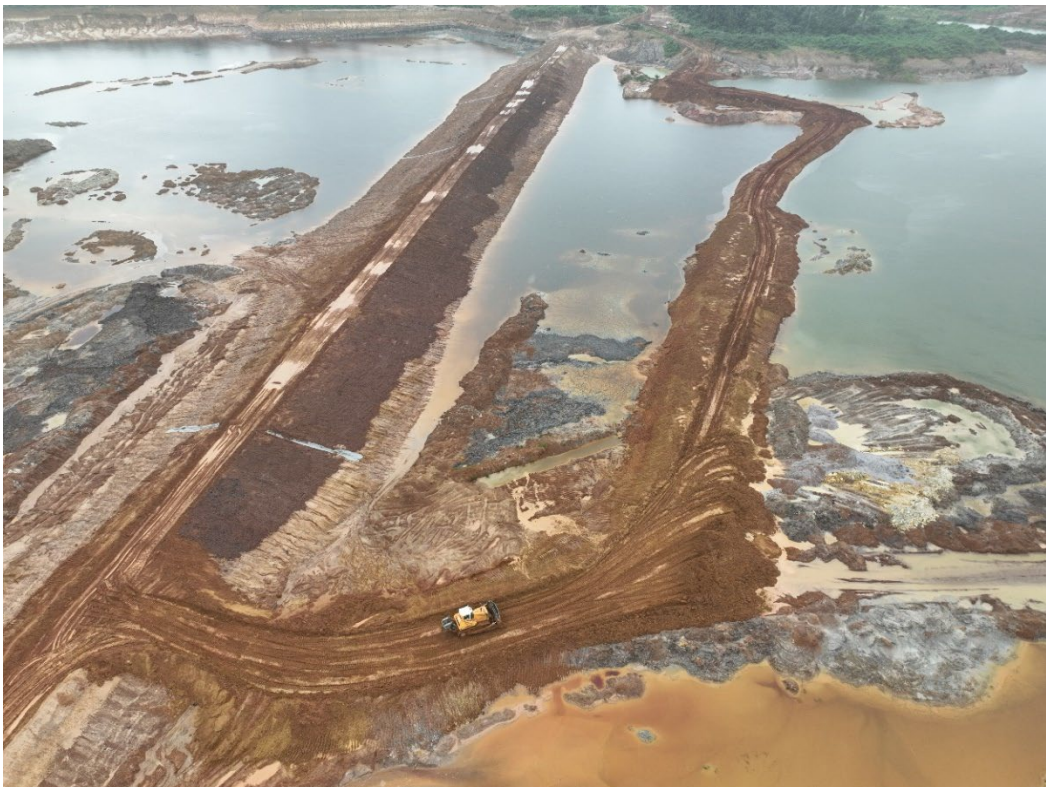
Gbeni In-Pit Wall Construction
