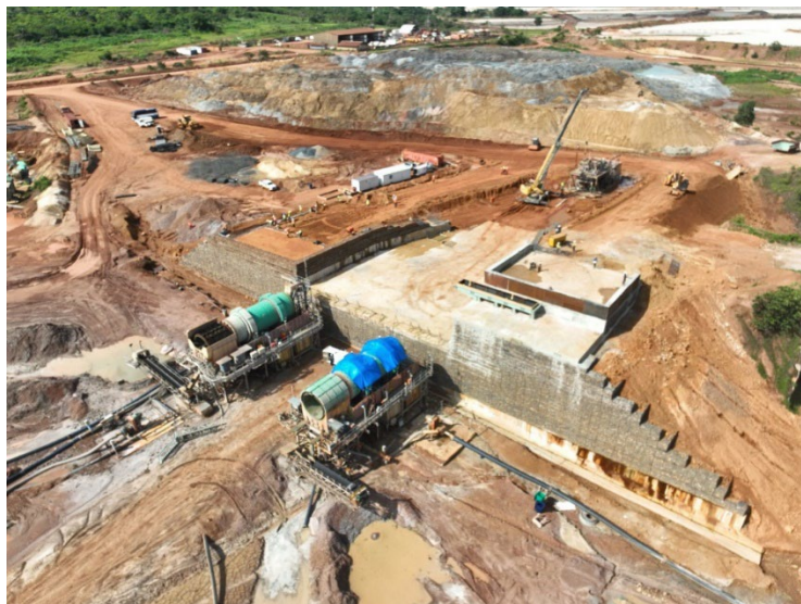
DM1/4 Gabion wall under construction with completed conveyer slab
